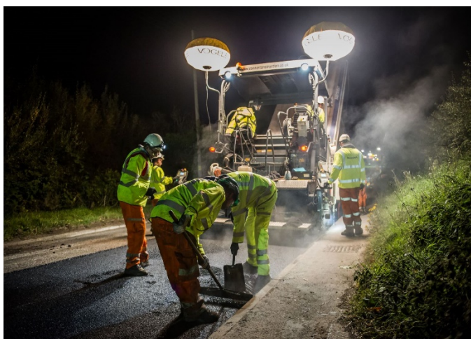
Figure 11: Highway Maintenance xiv
